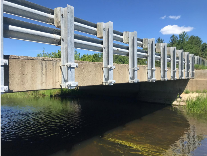
Document Name: IMG_2479.jpg Category: Elevation Span Number: Comments: East elevation
