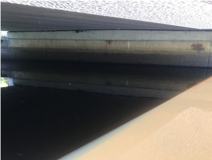
Document Name: IMG_2573.jpg Category: Substructure Span Number: Comments: South abutment
