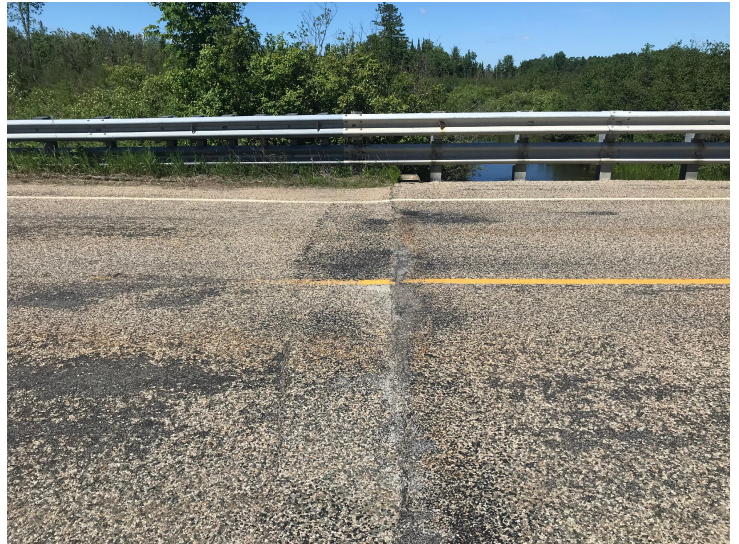
Document Name: IMG_2471.jpg Category: Joints Span Number: Comments: North reference line
