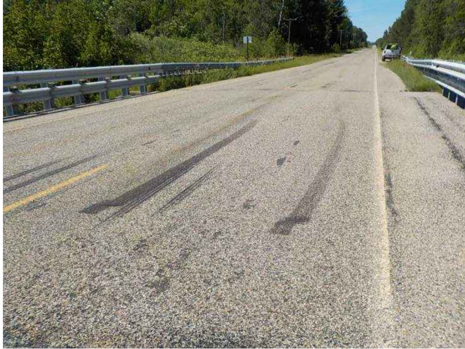
Looking across Keno Road Bridge
