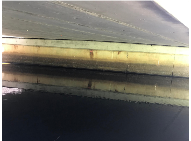
Document Name: IMG_2576.jpg Category: Substructure Span Number: Comments: North abutment
