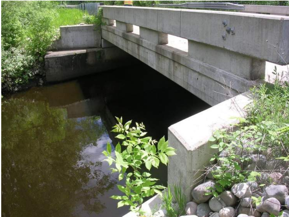
Fascia of Old US-27 Bridge
