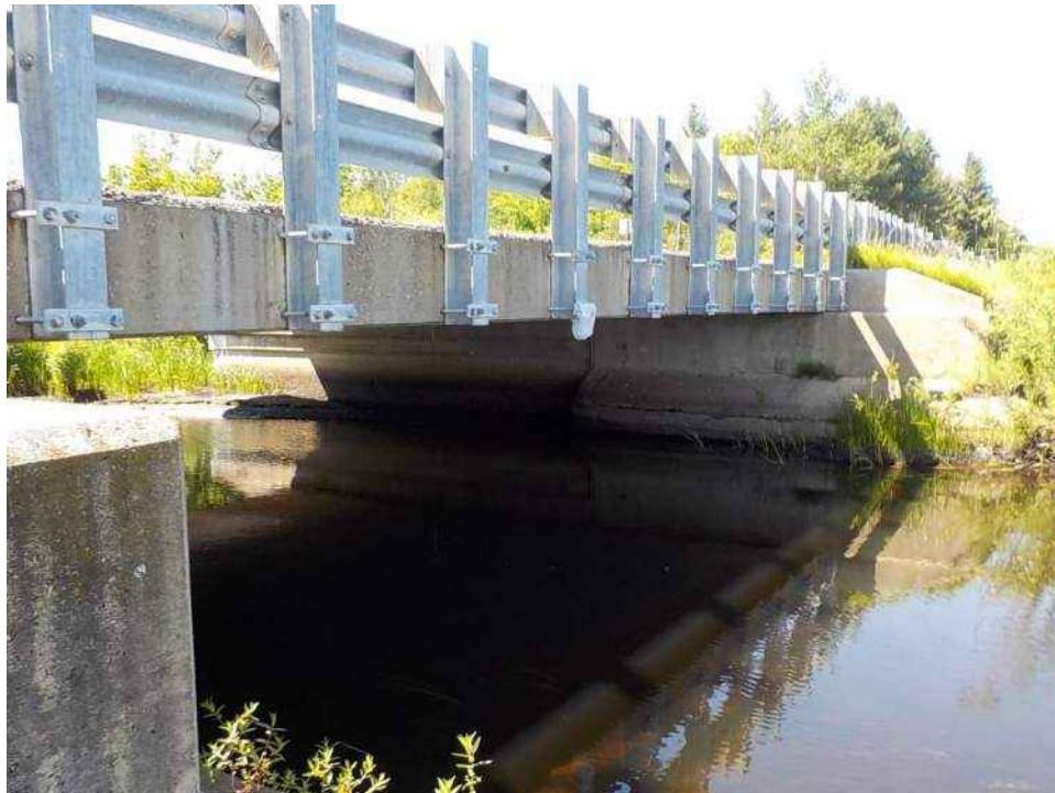
Fascia of Keno Road Bridge
