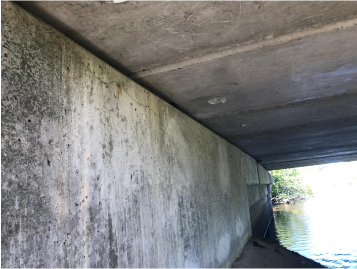
Document Name: IMG_2475.jpg Category: Substructure Span Number: Comments: South abutment
