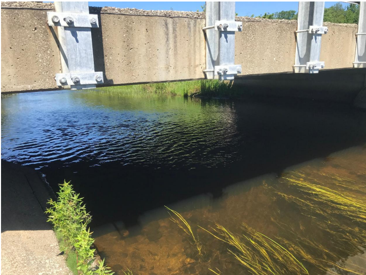
Document Name: IMG_2472.jpg Category: Superstructure Span Number: Comments: Precast beams
