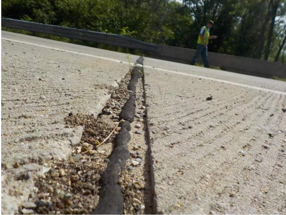
Joint at bridge approach
