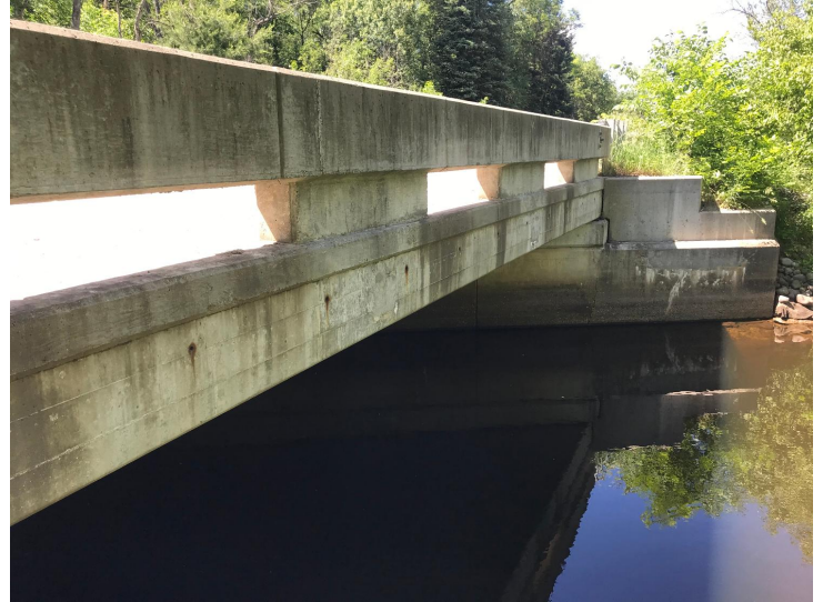
Document Name: IMG_2574.jpg Category: Elevation Span Number: Comments: East elevation
